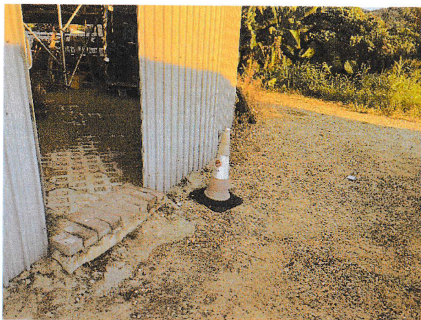
Photo no.4 As shown, the existing ground level of the proposed site is slightly higher than the outside village road.
