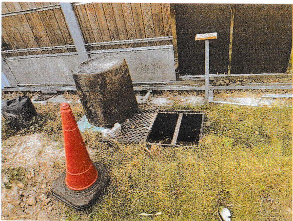
Photo no. 3 As indicated in the drainage layout plan there will be a proposed 225mm U-channel and two desilting pits to collect the stormwater that induced in the lots.
